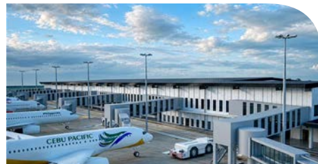
CATICLAN AIRPORT PASSENGER TERMINAL
