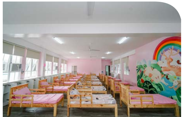
White Cross Facility Renovation San Juan, Metro Manila
