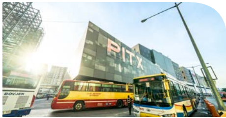
PARAÑAQUE INTEGRATED TERMINAL EXCHANGE (PITX)
