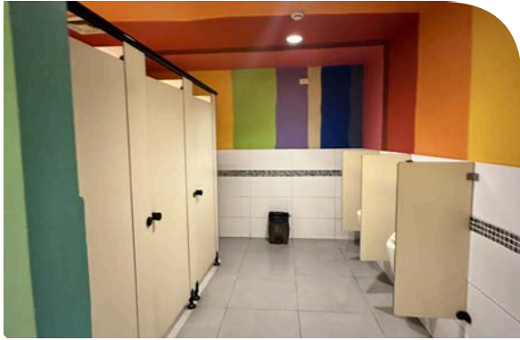
Museo Pambata Restrooms Renovation Roxas Boulevard, Metro Manila
