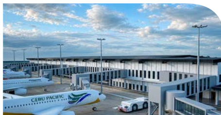
CATICLAN AIRPORT PASSENGER TERMINAL
