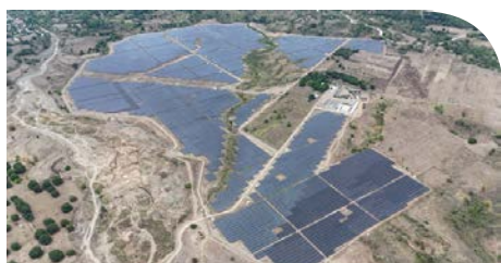
105MWP BINALONAN SOLAR POWER PLANT
