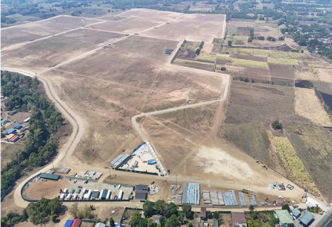
LUMBANGAN SOLAR POWER PLANT
