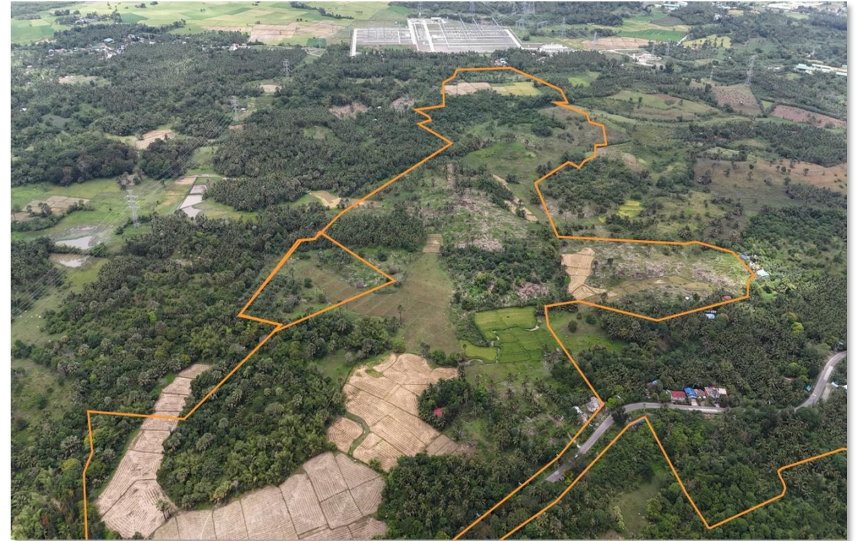
PAGBILAO SOLAR POWER PLANT
