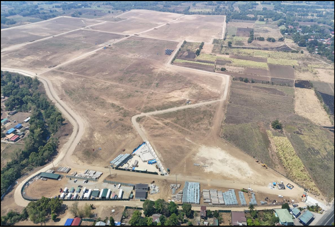
LUMBANGAN SOLAR POWER PLANT
