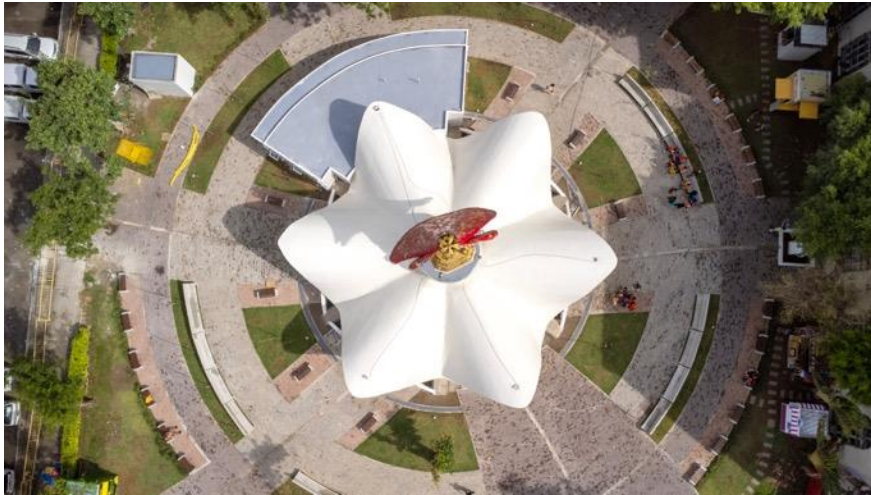
An aerial view of the chapel and surrounding park with some F&B kiosks
