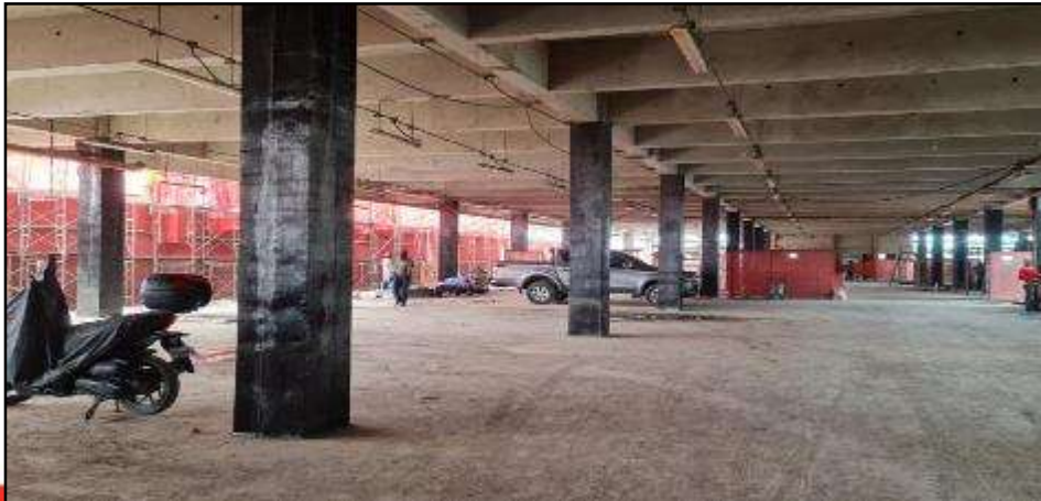
Carbon Fiber Reinforced Polymer Retrofitting Works at GF
