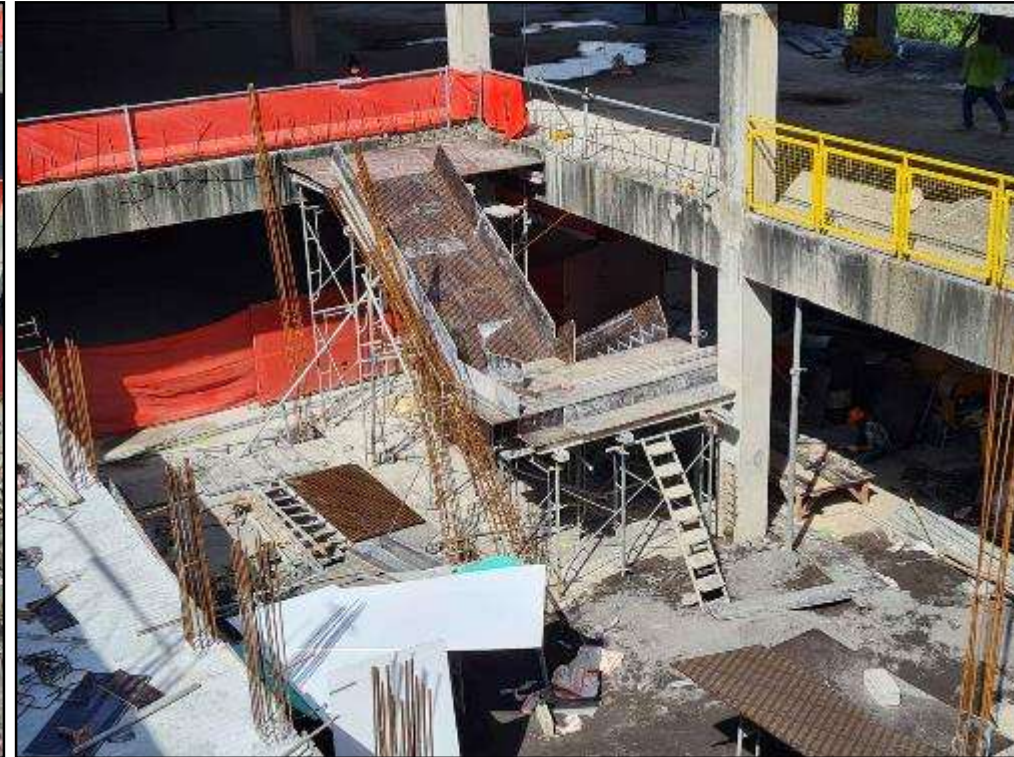
Stairs at Atrium Area
