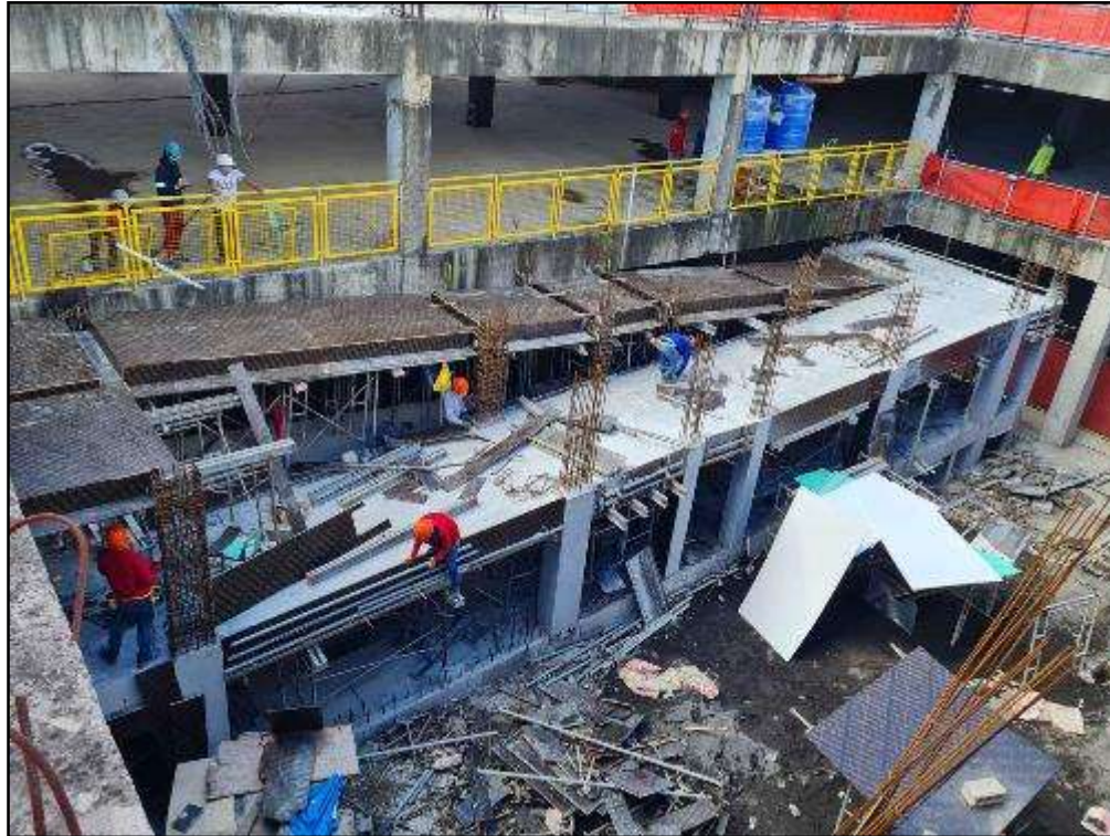
Ramp at Atrium Area
