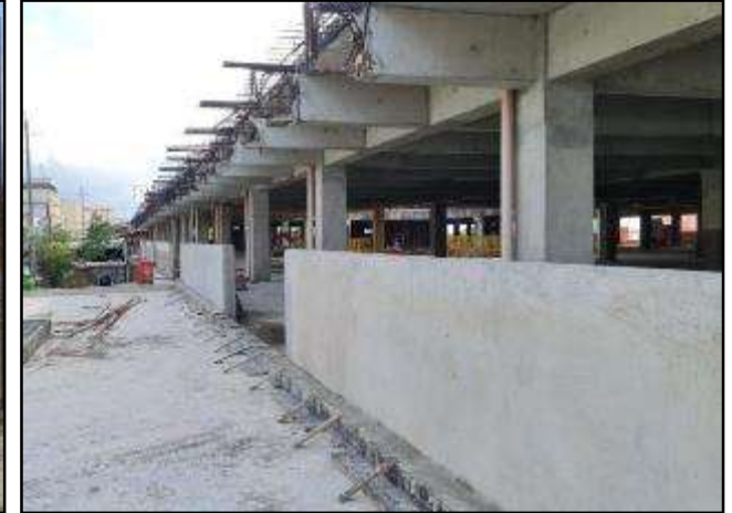
Parapet Wall at 3rdF along M.C Briones Street
