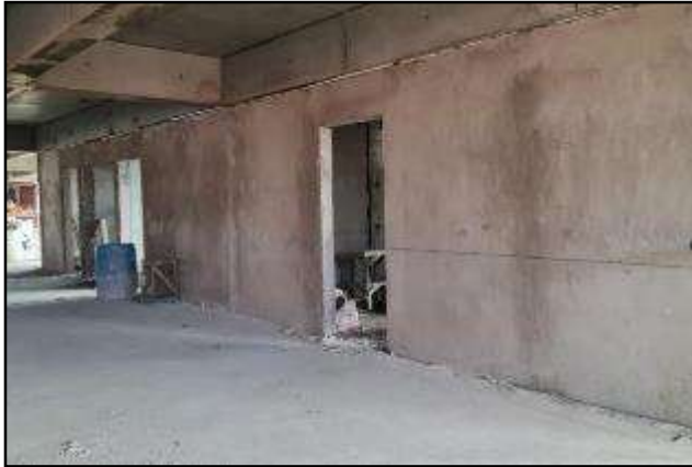
Toilet at 2ndF along Plaridel Street
