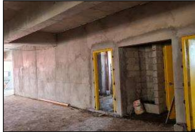
Toilet at 2ndF along F. Calderon Street
