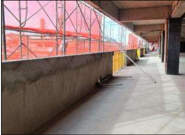
Parapet Wall at 2ndF along Quezon Blvd
