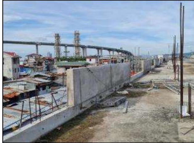
Parapet Wall at 3rdF along Quezon Blvd
