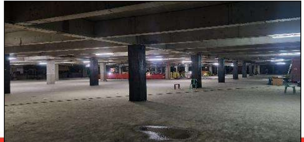
Carbon Fiber Reinforced Polymer Retrofitting Works at 2ndF
