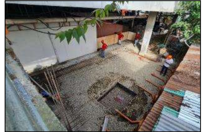
Toilet at Ground Floor along Plaridel Street
